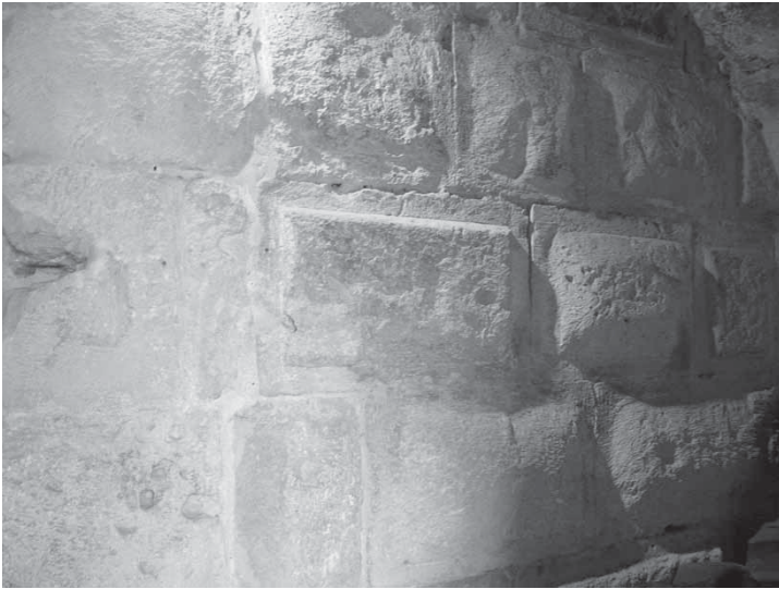
Fig. 12: Limassol Castle, north wall entrance, detail of marginally drafted masonry to the right of the portal [M. Olympios].
